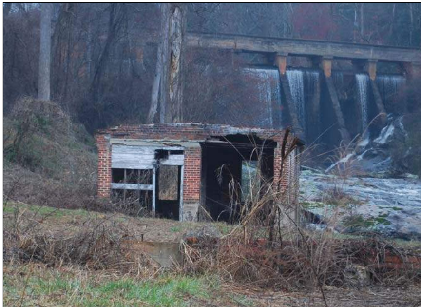
Photograph 21. Garage and Utility Building, facing northeast
