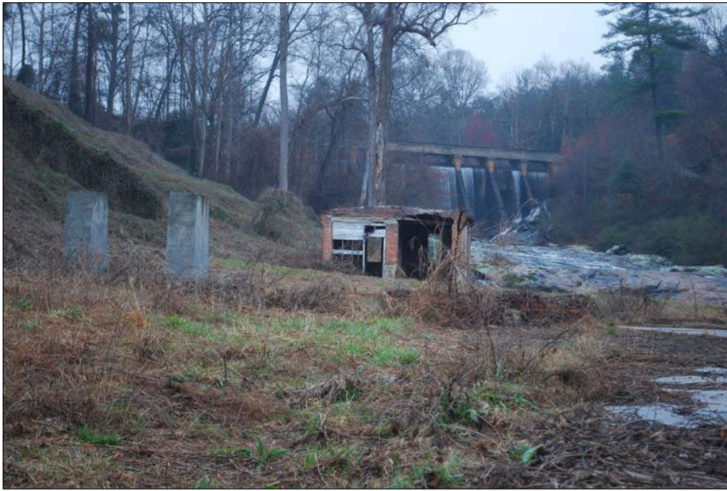
Photograph 7. View from Original Shuford Mills Complex toward Gunpowder Creek Dam, looking north
