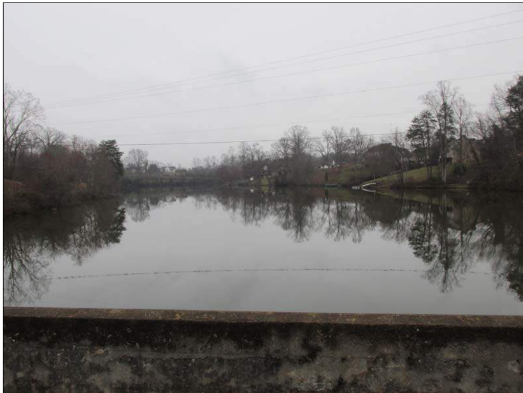
Photograph 4. Northwesternly View from Gunpowder Creek Dam toward Old Mill Pond
