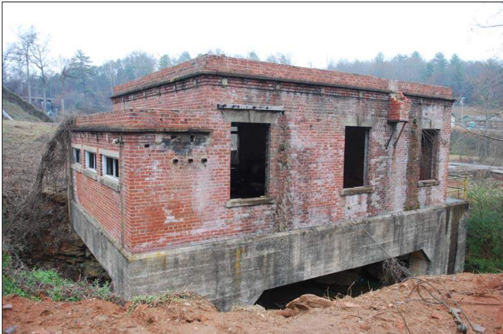
Photograph 6. Shuford Mills Power House, looking northeast
