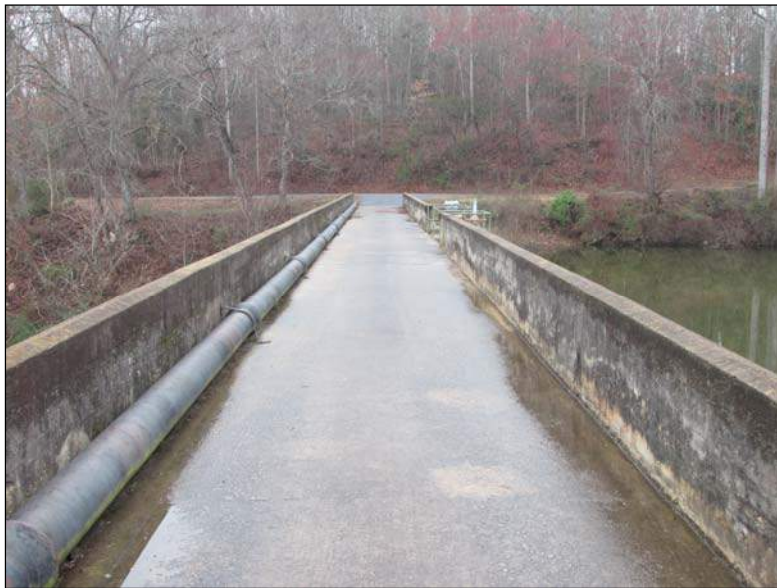
Photograph 17. Concrete Bridge across the Gunpowder Creek Dam, looking east
