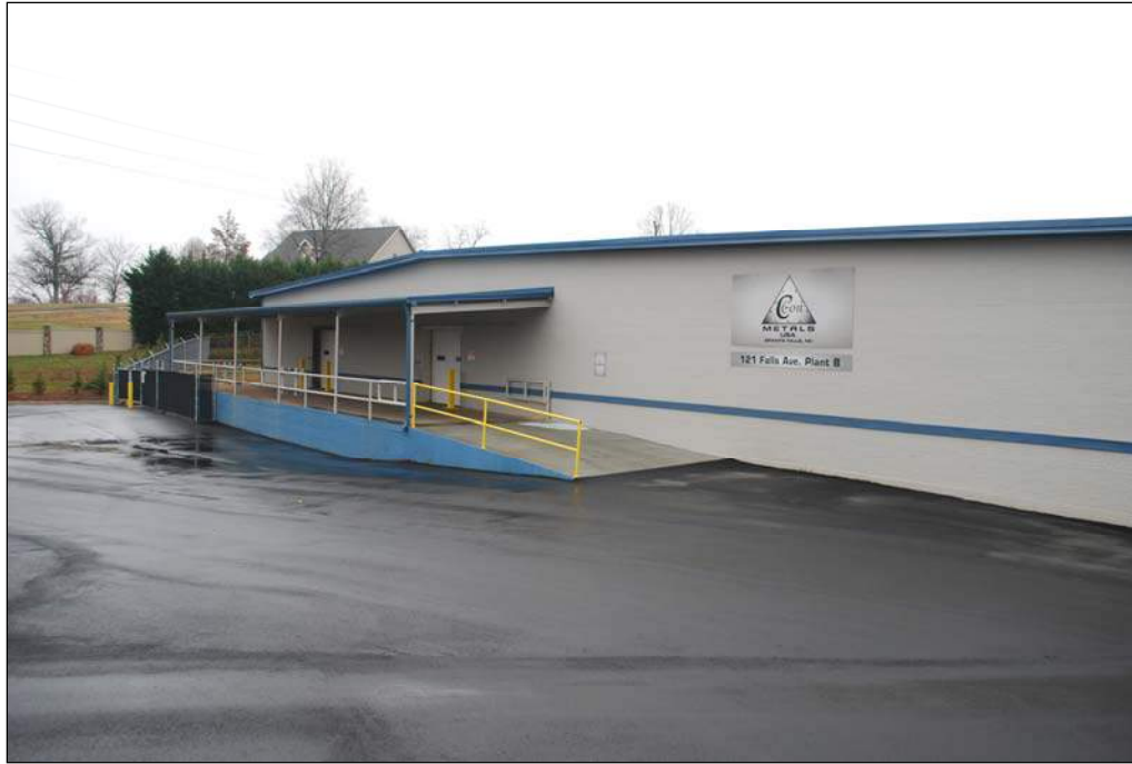
Photograph 1. Circa 1970 Plant Building Fronting Falls Avenue
