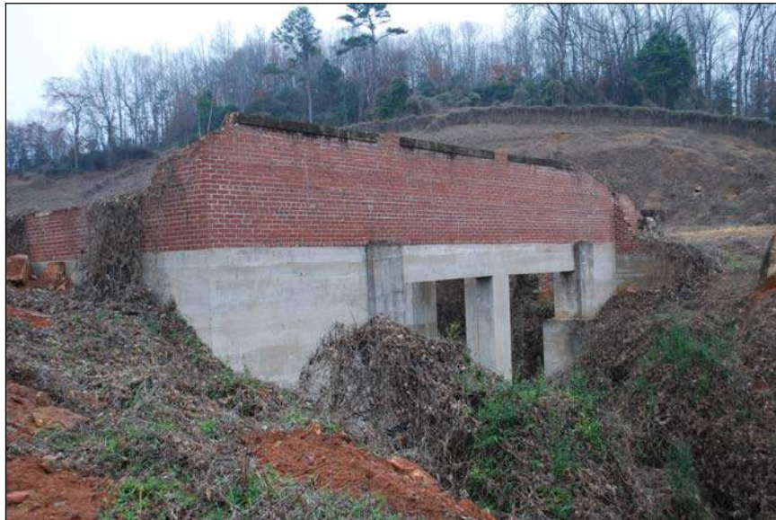
Photograph 19. Concrete Foundation and Brick walls of Plant No. 1, facing northwest
