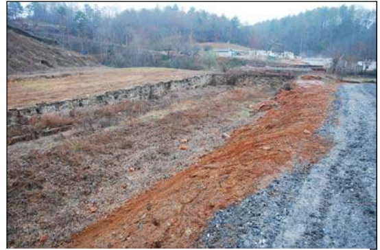
Photograph 18. Stone Foundation of Plant No. 1 (see Figure 4), facing east
