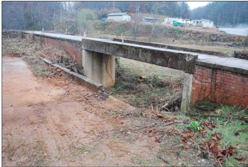
Photograph 20. Brick and Concrete Bridge Crossing Branch of Gunpowder Creek, facing northeast.
