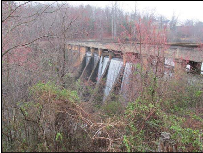
Photograph 16. South Side of Gunpowder Creek Dam, looking northeast
