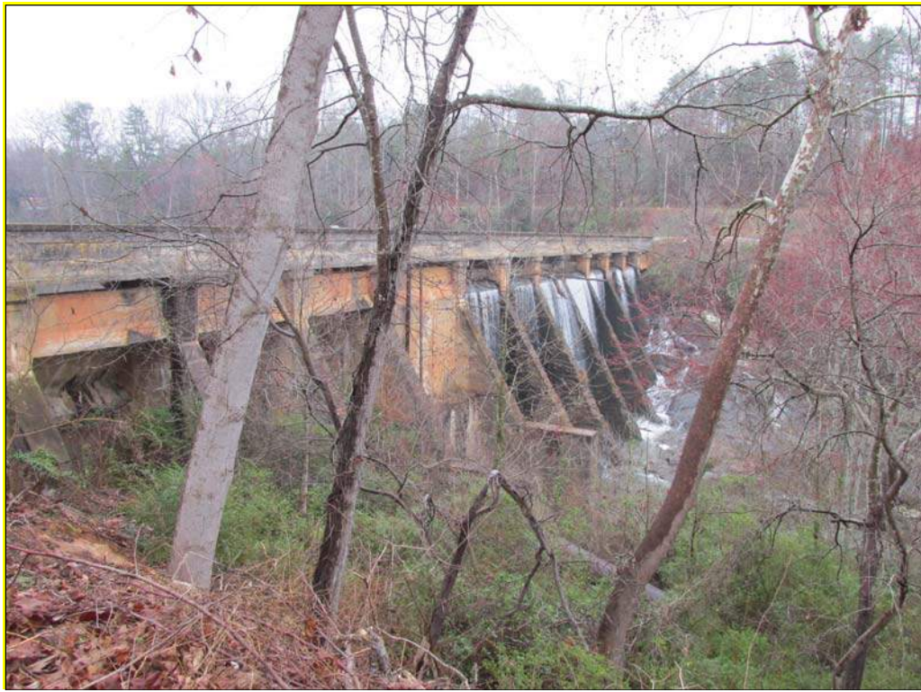
Photograph 3. Gunpowder Creek Dam, looking northeast
