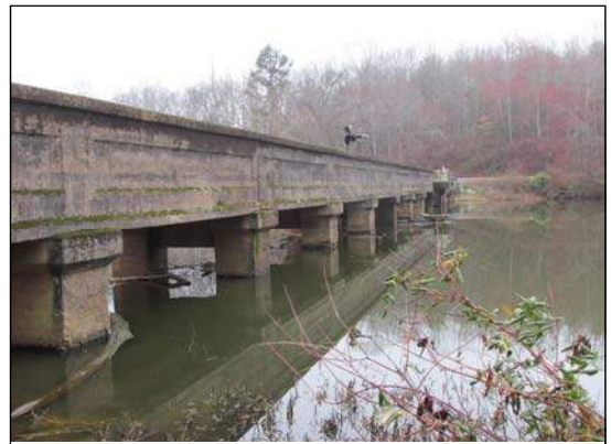
Photograph 15. Upstream Side (North) of Gunpowder Creek Dam, looking southeast
