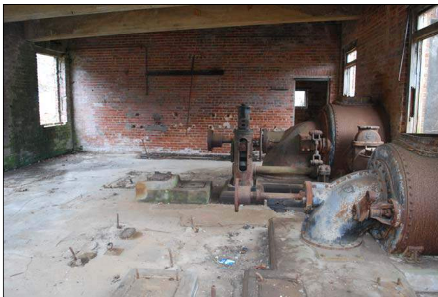
Photograph 23. Interior View of Power House
